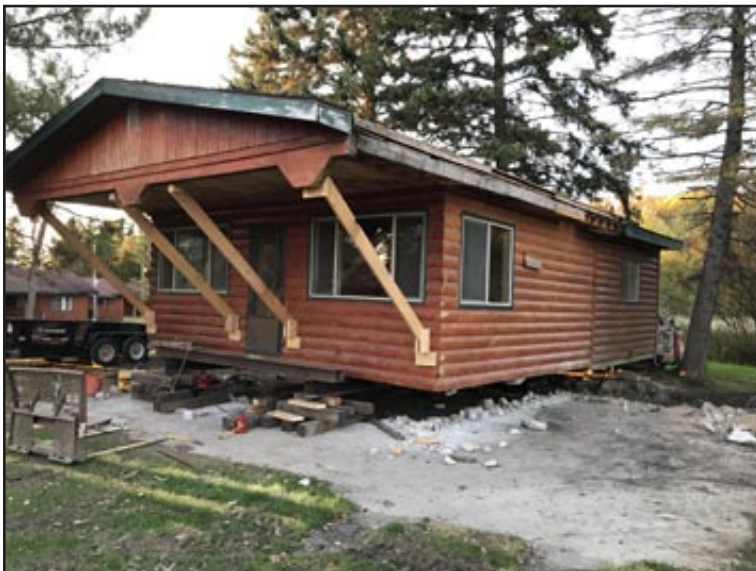
Old Cabin 9 is lifted and ready to be moved.
