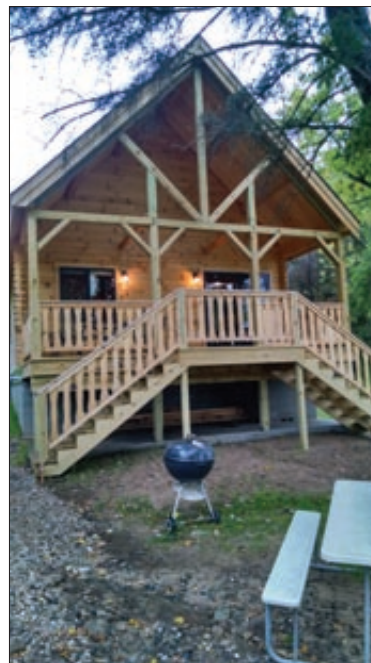
Two new cabins were completed from demolition to reservations in three months.
